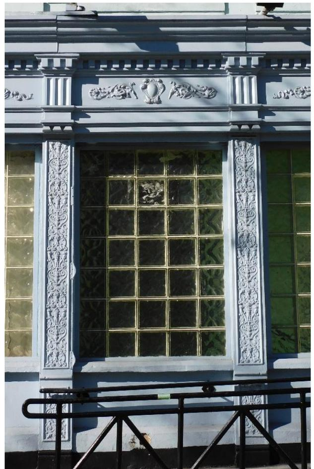
Figure 2: Detail of cast iron columns. Frieze is a likely replacement with a composite material (not magnetic).
