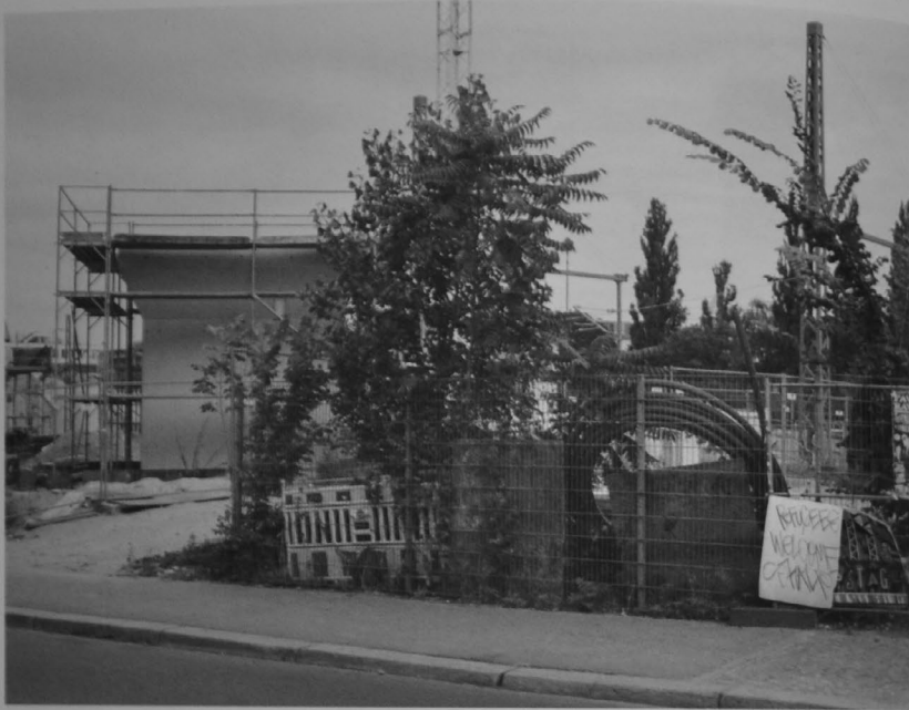
Construction site of infrastructural development of Deutsche Bahn AG at Ostkreuz
