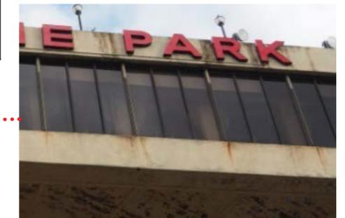
Corroding window frames that are staining the concrete
