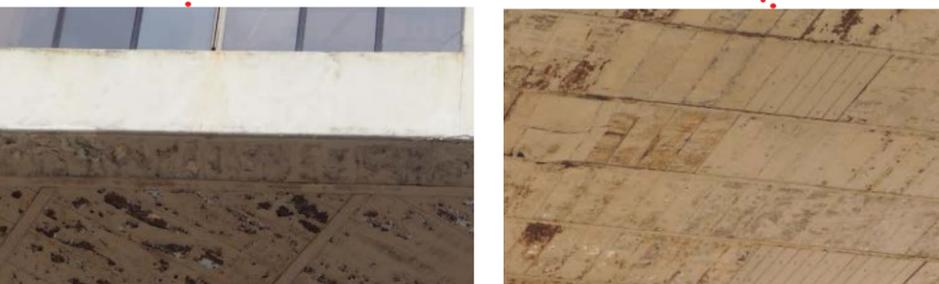
Peeling paint and rusting metal ceiling at the underside of the building
