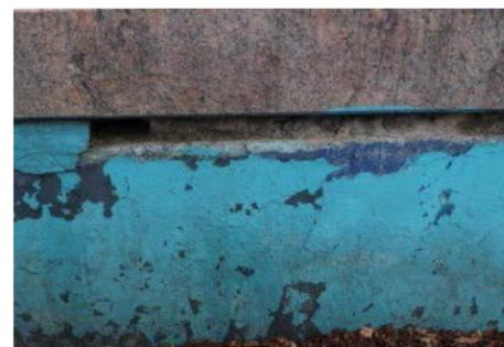
Loss of concrete bedding for the granite block
