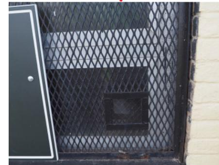
Replacement of the window with a non-homogeneous material
