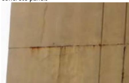
Rust that appears at the seam joints suggesting rusting of the metal anchor/sub-structure
