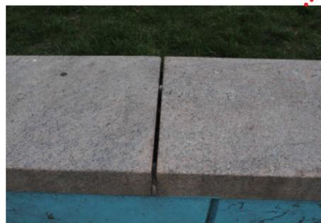
Loss of mortar in between the granite joints
