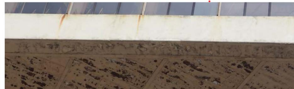
Blistering paints underneath the concrete panel due to water infiltration
