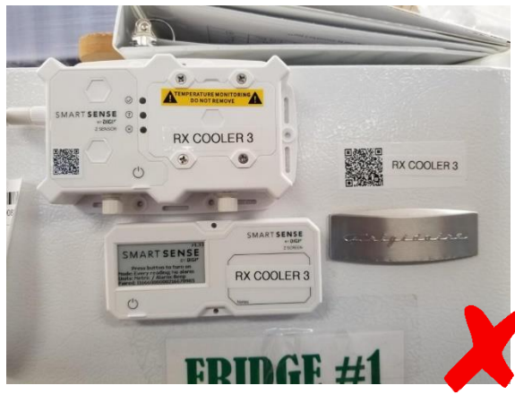
Figure 3.5b- Incorrect QR & ZSensor Placement for RX
