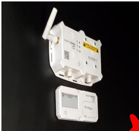
Figure 2.3a Incorrect FS Install
