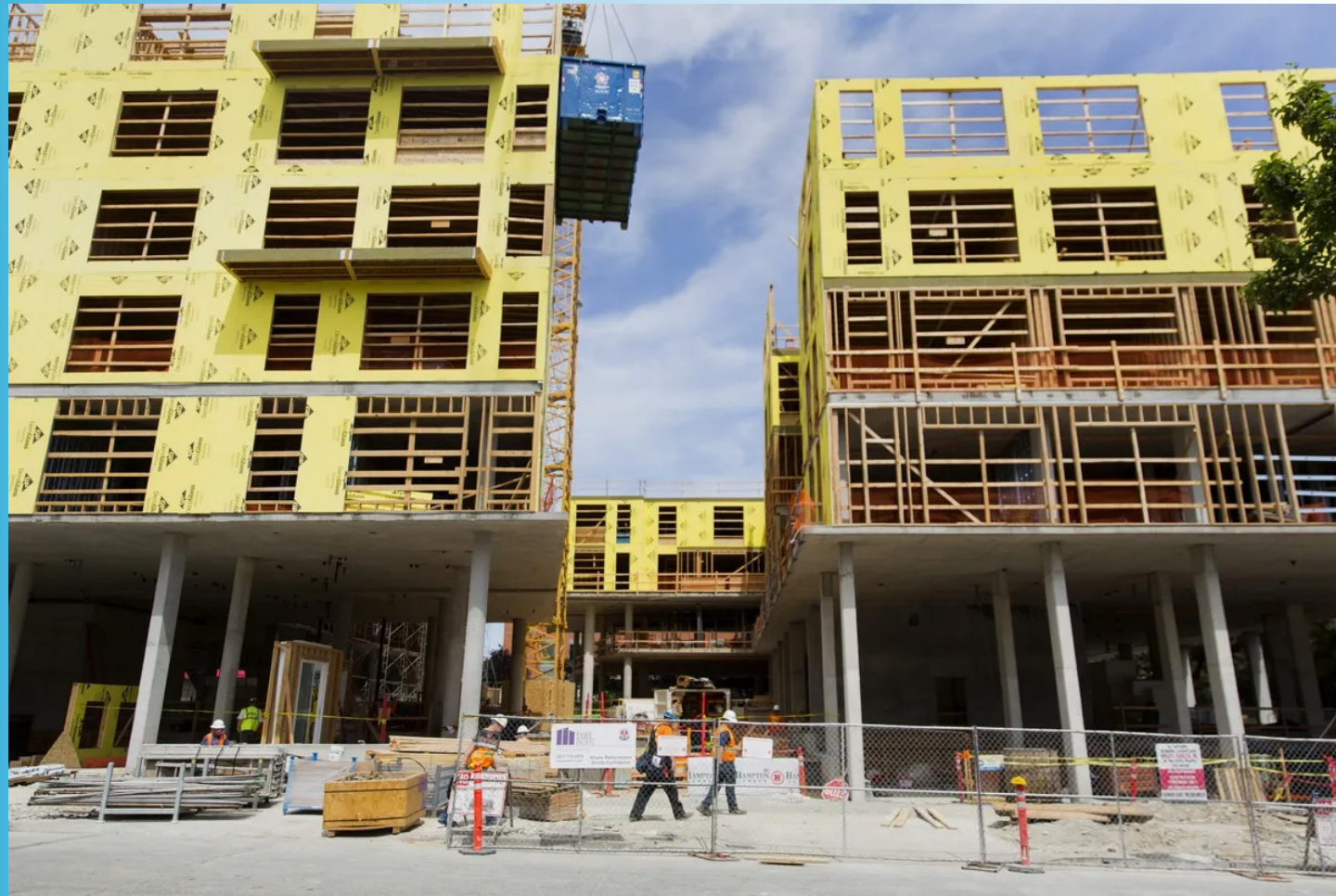
Apartment Construction in Seattle. Source: Bloomberg News
