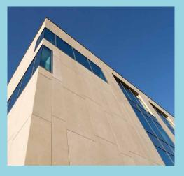
of the blonde sandstone used in the surrounding areas. Corners to the large box created by the cladding have a birds-mouth detail to create finer corners that define the building edges.
