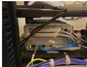
Figure A: Showing the BCM on System Rack Disconnect from port 1 (second from left)
