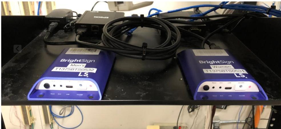
2. Unplug network cable from the Seneca DMP. BrightSign players will not have a network cable connected. **DO NOT UNPLUG Cat6A CABLE FROM THE EPSON TRANSMITTER as it provides the video signal to the projector on the sales floor.**
