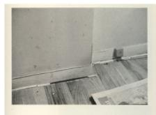
A TENANT TRIES TO KEEP OUT COCKROACHES BY FILL-ING THE AIRSPACE BETWEEN THE FLOOR AND MOLDING WITH PUTTY.
