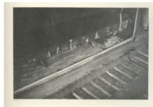
A VIEW OF SPACE UNDER THE HEATING UNIT WHERE CONCRETE HAS BEEN POURED BY THE TEN-ANT TO PREVENT THE ENTRACE OF RATS AND INSECTS.
