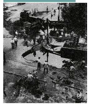
Water main burst in 1956 at Seventh Avenue and 145th Street under the toad causing a hole that was estimated 14' deep and 40' x 22' wide. Fear of fire due to lowered water pressure resulted in deployment of fire boats. The water burst also caused a critical water shortage throughout the area. The surrounding area is repeatedly affected with water supply shortage and public transportation suspended by water burst.
