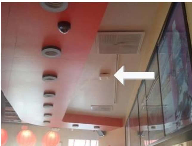
The WAP mounts to a bracket that is mounted to the ceiling
