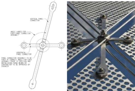
Fig. 6. Perforated infill panels and universal node assemblies with cruciform armatures and cable swages.
