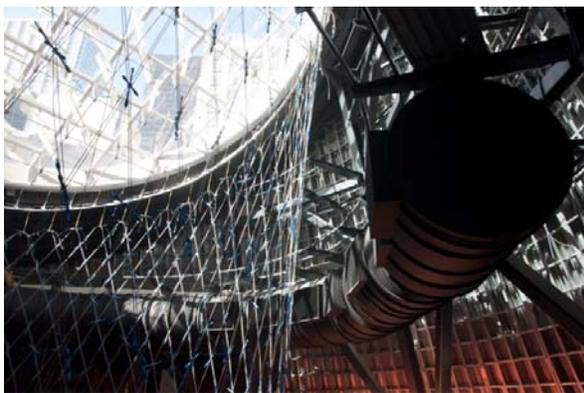
Fig. 7. Smoke intake ducts behind the net as seen during installation.
