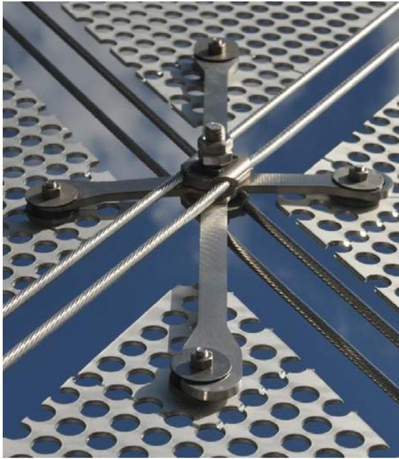
Fig. 3. Perforated infill panels and universal node assemblies, with cruciform armatures and cable swages.
