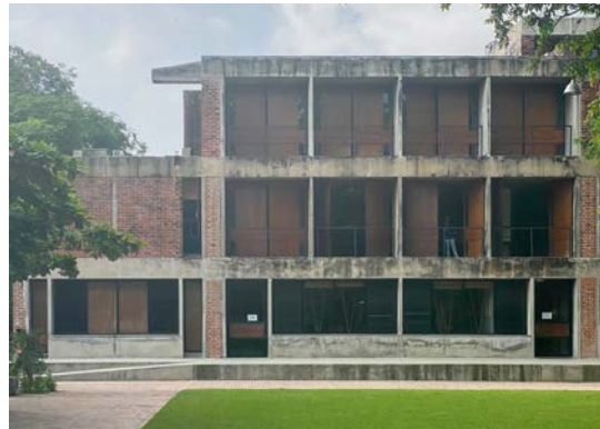
Brick walls and concrete frames with operable wood doors.
