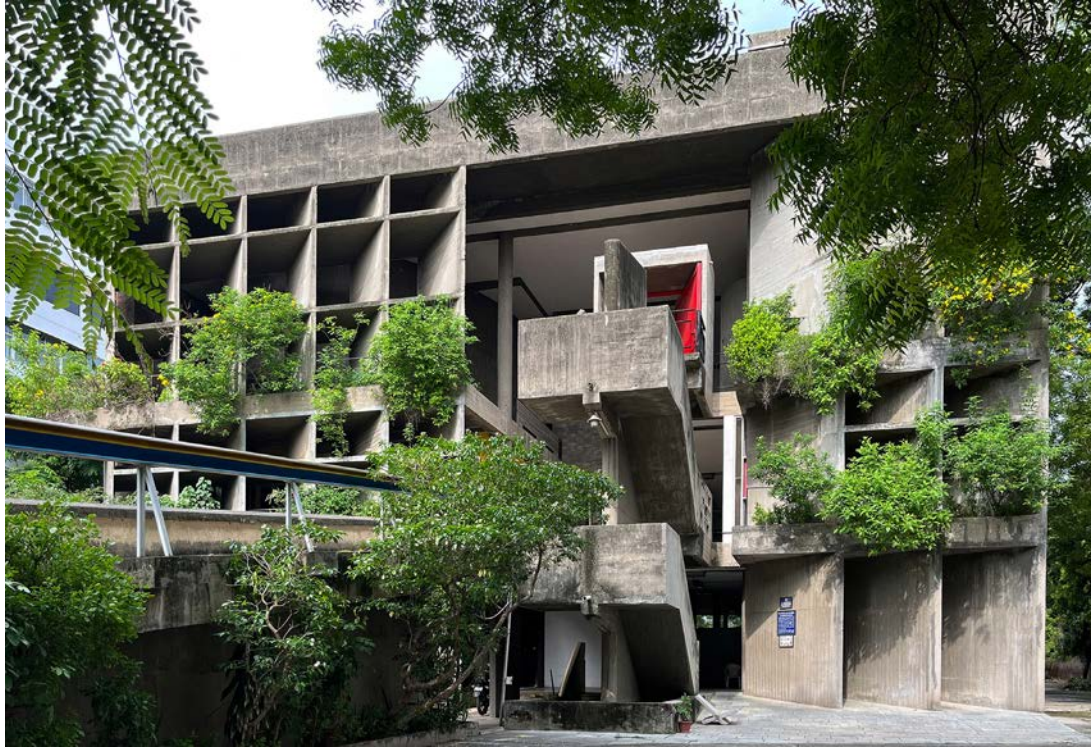
Brise-Soleil on West Façade next to ramp (Ph. Allon Morgan).
