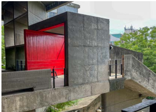
Large pivoting door on second floor at stair's landing.
