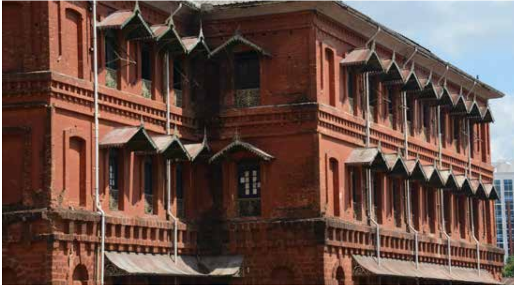
FIGURE 13. Former Myanmar Railways Headquarters building in Yangon
