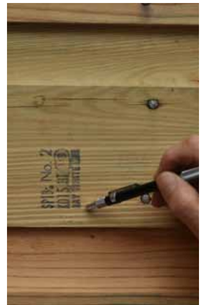
FIGURE 126 Owner and architect Gilbert Mangones explaining the restoration work he is doing on his house at 24 Avenue Lamartiniere, shown in Figures 1.18 and 1.23. The new ship-lap siding is pressure treated imported timber. The timber grade stamp is shown above.
