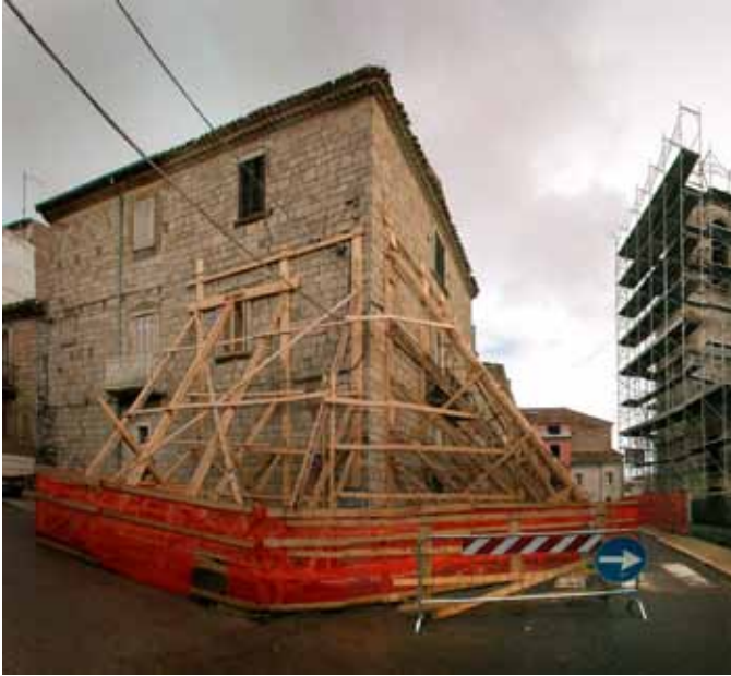
FIGURE 121 Examples of shoring in Italy after the Molise earthquake, showing the heavier timber diagonal braces in the example on the left, and polypropylene straps holding the building together on the right.
