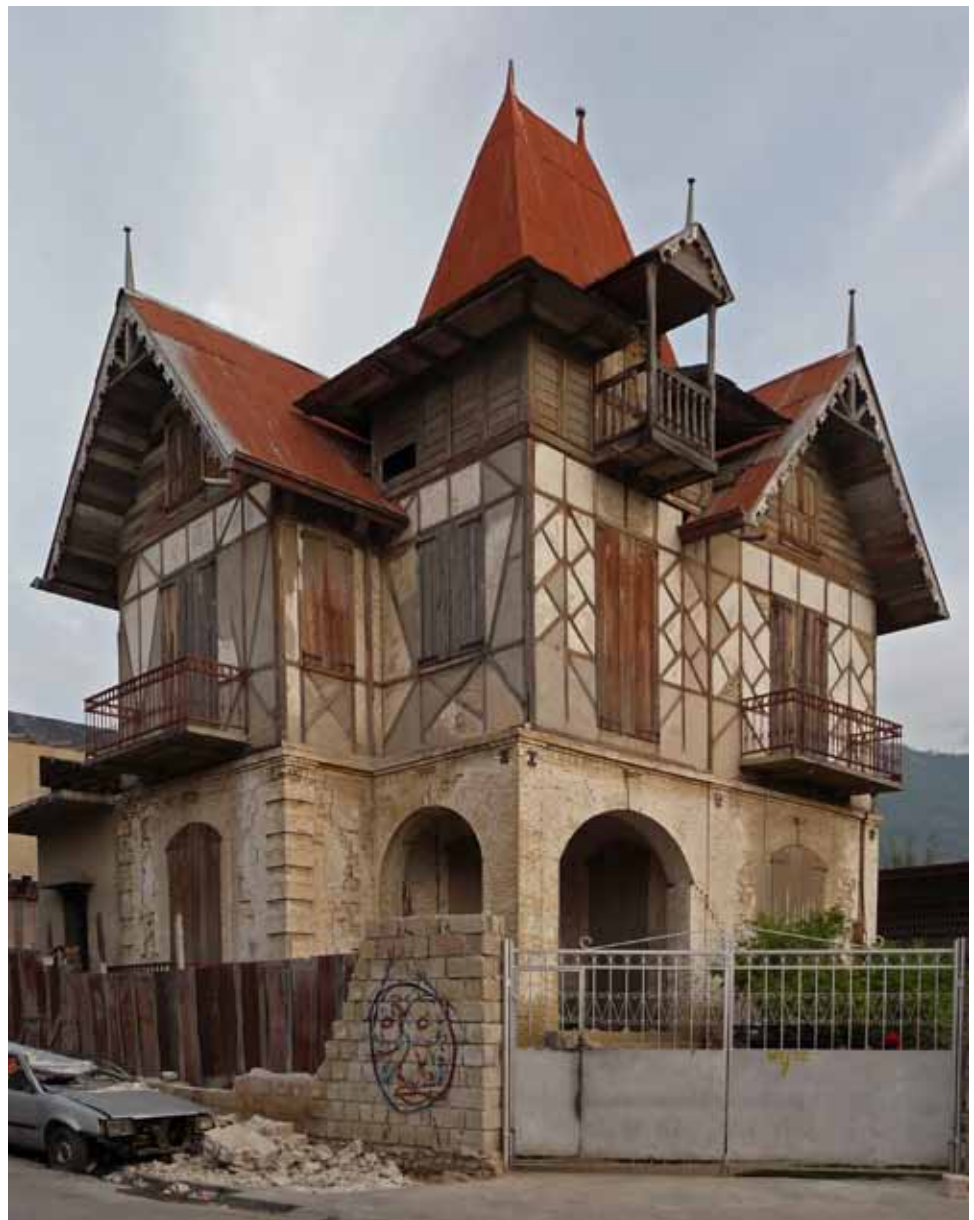
FIGURE 49 Hybrids are very common. This Gingerbread house at 59 Lavaud 3 utilizes all three wall-construction systems: Attic walls—wood frame Second story—colombage First story—masonry bearing wall Note also the one-story concrete addition at the back left corner.
