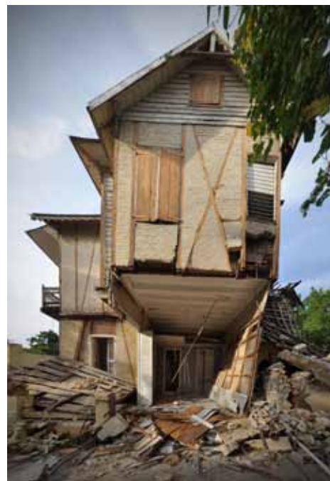
FIGURE 137 left: House on Rue Jose Marti where the concrete addition collapsed, leaving the Gingerbread house cantilevered over the rubble. Right: The son of the owner of this house is pointing to the place where his brother remains buried in the rubble of the collapsed concrete addition.
