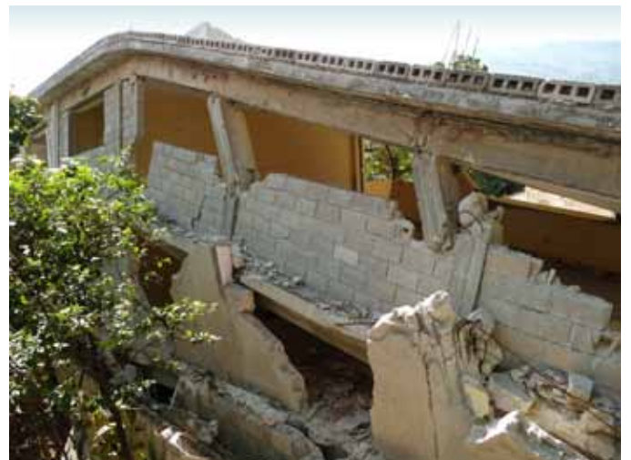
FIGURE 113 Owner of Rue 5 Jose Marti points to adjacent collapsed concrete and concrete block school building.
