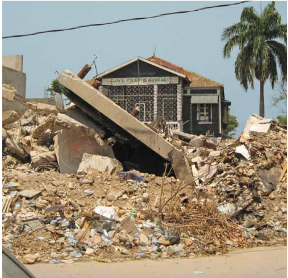
FIGURE 118 In a typical scene, a Gingerbread stands intact beyond the tragic collapse of a modern concrete building
