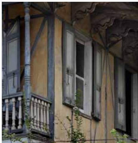
FIGURE 44 House at 15 Rue M showing undamaged second floor panels coated with a colored whitewash, giving an attractive patina to the surface of the stucco.
