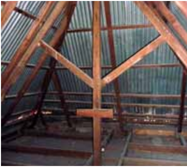
FIGURE 54 Corrugated steel roof with braced roof framing.
