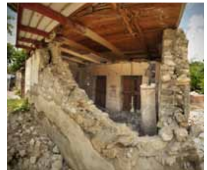
FIGURE 98 House in Léogâne where the solid rubble stone wall on one side partially collapsed, while the side with the two door openings with brick piers and rubble panels seen through the collapse remained standing with much less damage.
