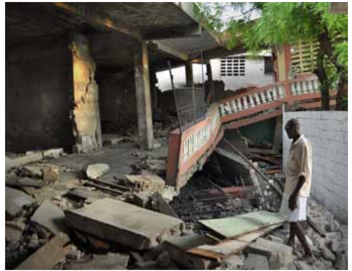
FIGURE 112 A small colombage school building at 16 Lamartiniere which had a two-story addition behind it. This addition collapsed completely, but the original building is still intact and in use.
