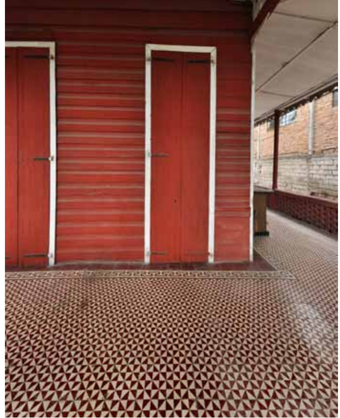
FIGURE 34 The house at 24 Avenue Lamartiniere, showing the characteristic ship-lap siding and simple undecorated doors, with an ornate tile surface on the lower porch.
