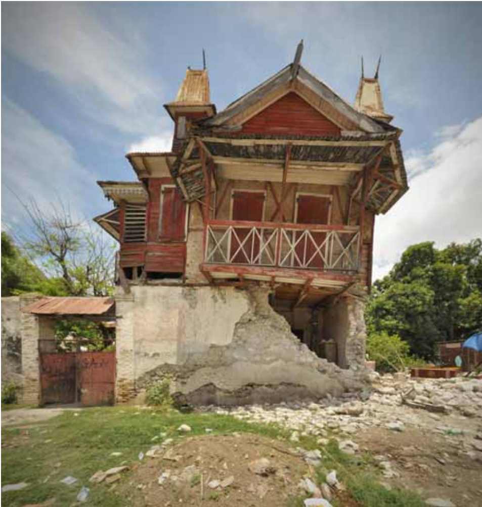
FIGURE 98 House in Léogâne where the solid rubble stone wall on one side partially collapsed, while the side with the two door openings with brick piers and rubble panels seen through the collapse remained standing with much less damage.
