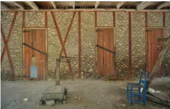
FIGURE 25 left: A barn in Léogâne is an example of rubble stone colombage made with stronger igneous rocks than those used in Port-au-Prince, and not stuccoed. right: A heavily damaged colombage wall showing the rubble stone infill characteristic of Port-au-Prince.
