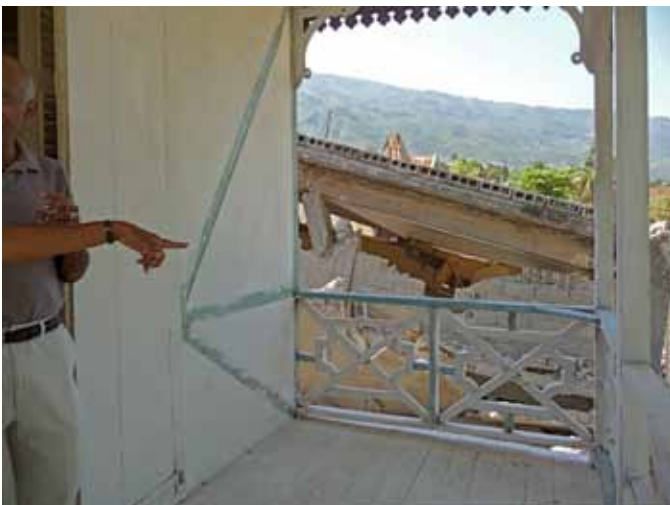
FIGURE 113 Owner of Rue 5 Jose Marti points to adjacent collapsed concrete and concrete block school building.
