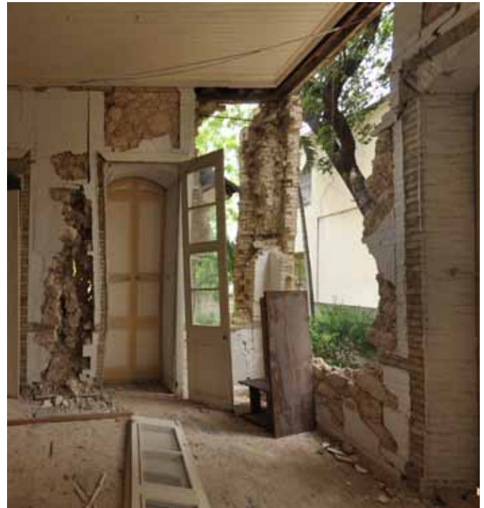
FIGURE 95 above left The Dufort House showing the collapse of the rubble panels, leaving the piers standing holding up the almost undamaged upper floor structure. The remarkably large pile in front shows the volume of rubble masonry removed from the house after it had collapsed. above right The interior of the Dufort House, also shown in Figure 77, showing how the collapse of the rubble panels left the house standing on the brick piers which were left like free standing columns. left This house also had steel or wrought iron reinforcing chains made up of rods hooked together for the full length of the exterior and major interior walls. In this case, rather than exterior plates to hold them, their wall anchors were imbedded under the outer wythe of masonry. The rods are also visible where they intersect at the corner pier that is still standing.
