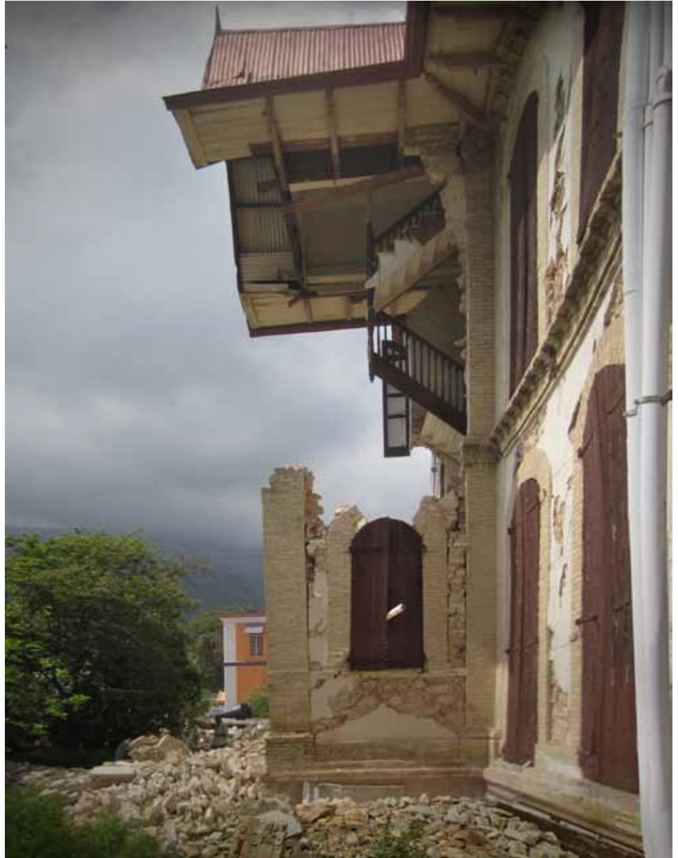
FIGURE 130 below left: Le Manoir on Avenue John Brown showing a heavy level of disruption of the masonry walls caused by the rapid degradation of the rubble stone panels during the earthquake. below right: A rubble panel on the second floor of the Villa Castel Fleuri that collapsed showing the displacement of the bottom of the brick pier into the doorway which resulted from the expansion forces from the panel.
