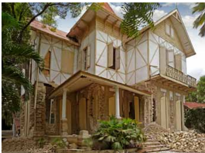
FIGURE 75 A pancaked concrete-frame building on the right and a colombage house on the left showing the comparative performance of these building types in a seismic event.
