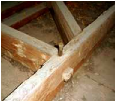
FIGURE 53 Attic framing with mortise-and-tenon joinery with wooden peg.
