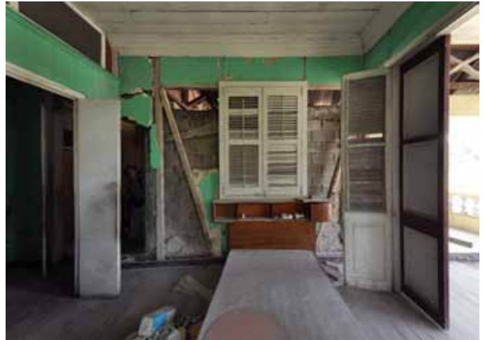
FIGURE 109 Interior and exterior of 51 Avenue Christophe showing reinforced concrete addition to the timber and colombage house. The two parts pulled away from each other during the earthquake.
