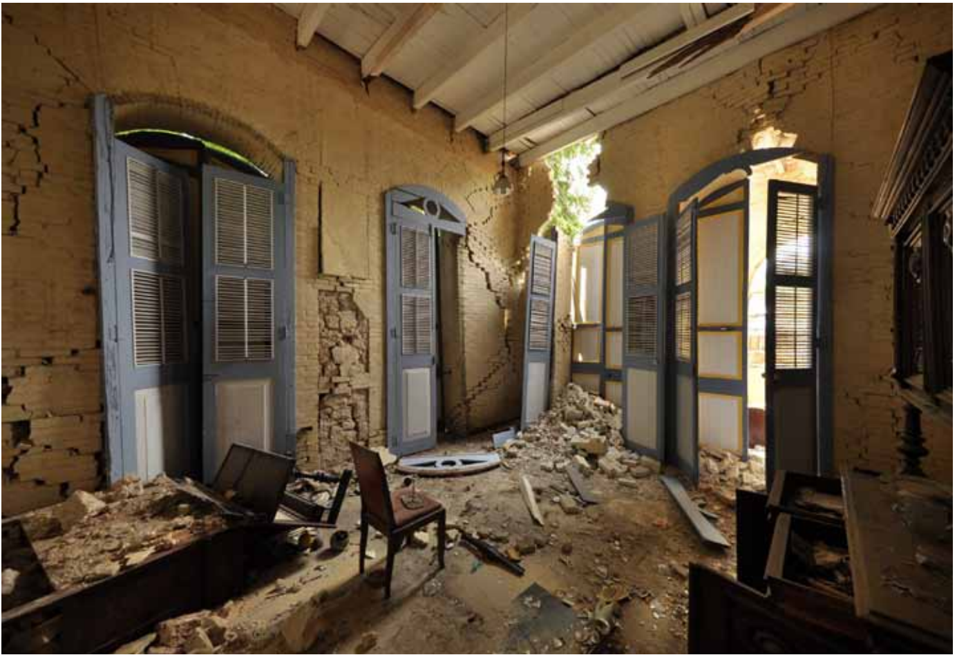
FIGURE 97 Two-story masonry house at 46 Avenue Christophe. During the earthquake, part of the second floor collapsed, followed by the subsequent collapse of the rest of the second floor. These photos show the ground floor, which remained standing, but with major rupture to the masonry walls, particularly at the corners. Right, the iron rod that had held the building together at the floor level is visible where it had failed because of corrosion. This image also reveals how the inner wythe of brickwork was not bonded to the outer layers of rubble stone. To form the inner corner of the room there is a layer of brick, whereas in the middle of the room, the rubble stone panel goes through the entire thickness of the wall.
