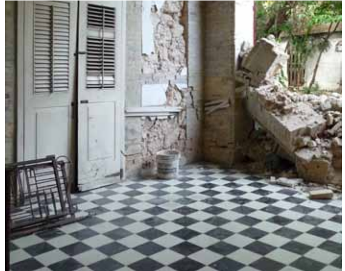
FIGURE 60 Tile over slab on grade at 5 Lavaud r.
