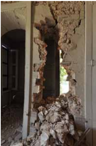
FIGURE 130 below left: Le Manoir on Avenue John Brown showing a heavy level of disruption of the masonry walls caused by the rapid degradation of the rubble stone panels during the earthquake. below right: A rubble panel on the second floor of the Villa Castel Fleuri that collapsed showing the displacement of the bottom of the brick pier into the doorway which resulted from the expansion forces from the panel.
