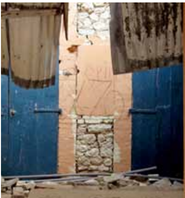
FIGURE 46 Characteristic 'brick frame' with rubble infill construction
