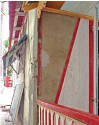
FIGURE 135 Well-intentioned but improper repairs with cement mortar in brick work ( left and center ), and cement plaster for colombage infill ( right ). Lime mortar and lime plaster should be used.
