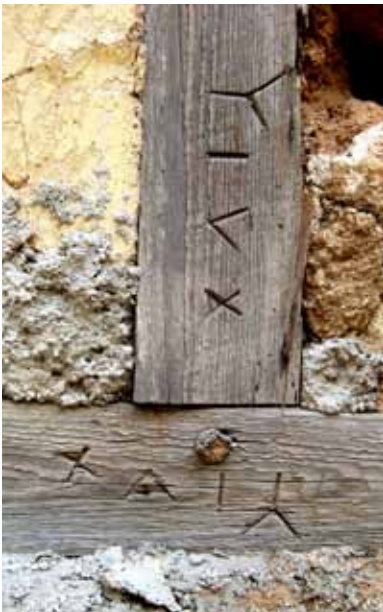
FIGURE 37 A detail of colombage construction. The wood frame is pegged with a trenail and the panel voids are filled with stone and lime mortar. The fill on the left still has the clay stucco in place. Note the carpenter's marks carved into the wood members.
