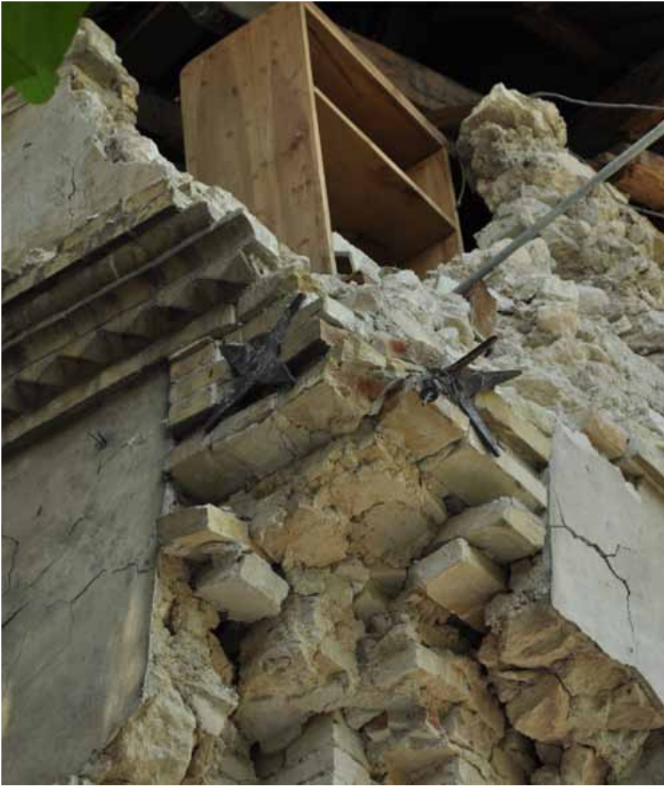
FIGURE 101: Iron chains are common in many of the masonry walls of the Port-au-Prince Gingerbread houses. Above is the first section of the chain with the star-shaped metal plate, and the view at left shows the metal plates where they remain holding the wall at the floor level in place, thus stopping the further separation of the walls at the corner. Had these floor level reinforcement rings not been installed, the lower floor walls would probably have collapsed as well.
