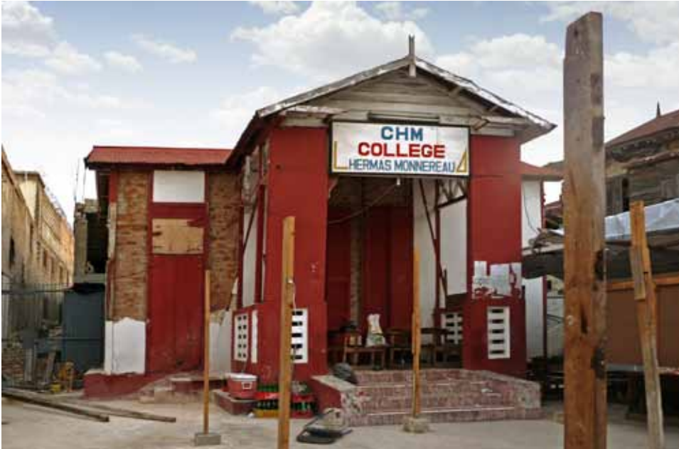
FIGURE 112 A small colombage school building at 16 Lamartiniere which had a two-story addition behind it. This addition collapsed completely, but the original building is still intact and in use.
