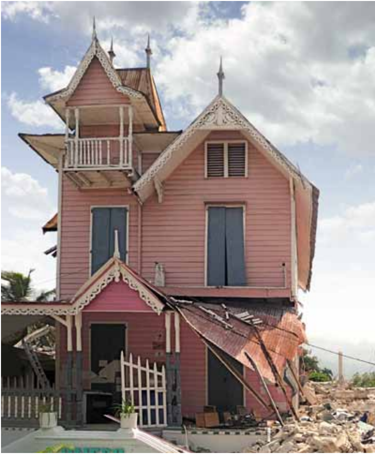
FIGURE 82 Wood frame Gingerbread at the Episcopal University on Rue Capois next to the site of a collapsed concrete building.
