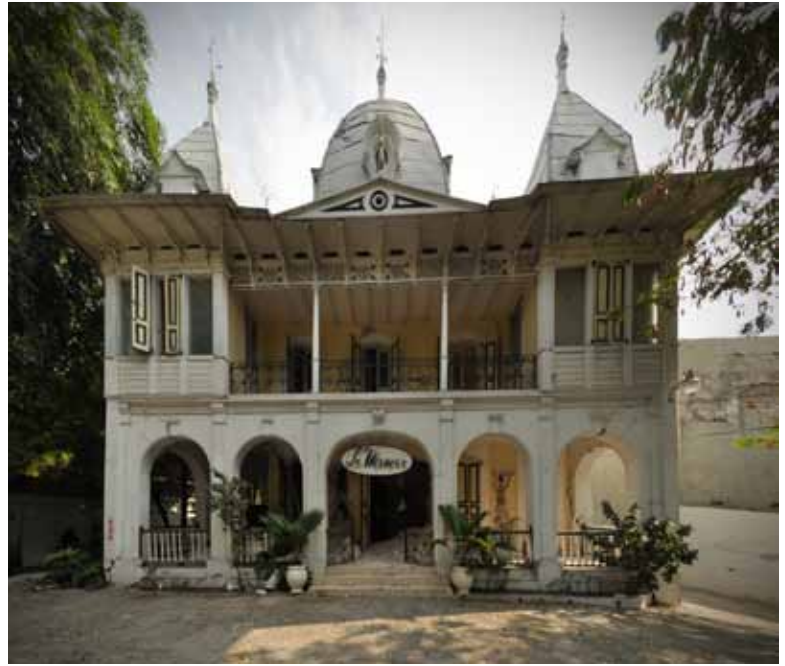
FIGURE 96 top : Exterior view of Le Manoir on Avenue John Brown. middle : interior view of Le Manoir showing a fully disrupted ground-floor wall where the rubble panels have collapsed, but the buildings remained standing on the brick piers. (view is a mosaic of several photos connected together). bottom : House at 65 Avenue N showing infill panels manifesting the onset of damage, but little displacement during the earthquake.
