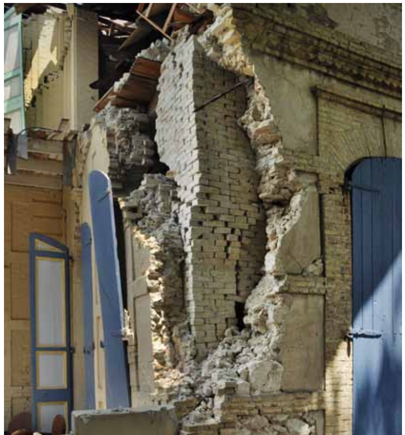
FIGURE 97 Two-story masonry house at 46 Avenue Christophe. During the earthquake, part of the second floor collapsed, followed by the subsequent collapse of the rest of the second floor. These photos show the ground floor, which remained standing, but with major rupture to the masonry walls, particularly at the corners. Right, the iron rod that had held the building together at the floor level is visible where it had failed because of corrosion. This image also reveals how the inner wythe of brickwork was not bonded to the outer layers of rubble stone. To form the inner corner of the room there is a layer of brick, whereas in the middle of the room, the rubble stone panel goes through the entire thickness of the wall.
