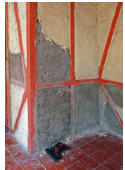
FIGURE 74 Improper repair of stone infill of colomage using cement mortar. These repairs would render a fill that was much harder and solid than the fill that it replaced.
