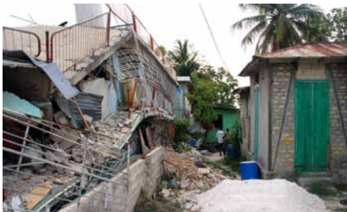
FIGURE 75 A pancaked concrete-frame building on the right and a colombage house on the left showing the comparative performance of these building types in a seismic event.
