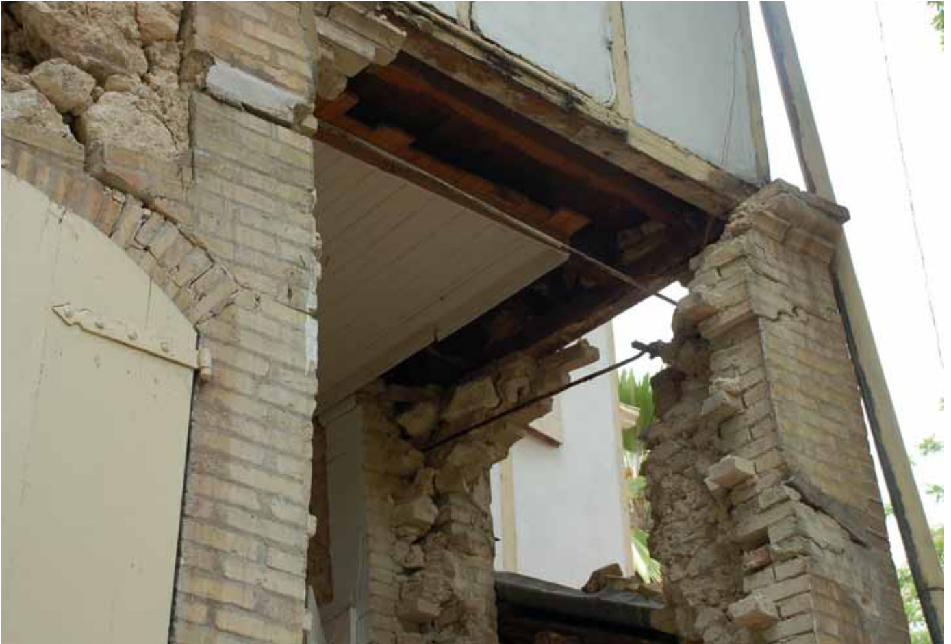
FIGURE 93 The masonry bearing walls of the ground floor of this Gingerbread are significantly damaged and partially collapsed, while the wood framed second floor remained almost undamaged.
