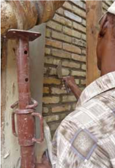
FIGURE 135 Well-intentioned but improper repairs with cement mortar in brick work ( left and center ), and cement plaster for colombage infill ( right ). Lime mortar and lime plaster should be used.
