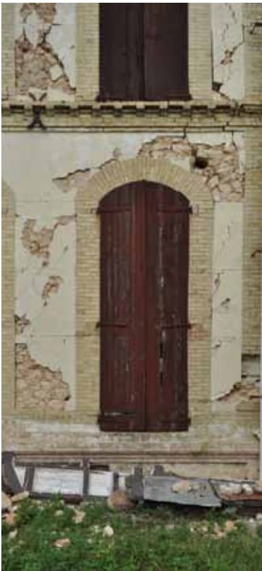
FIGURE 127 Typical 'brick frame' with rubble infill construction. Note crack pattern/energy absorption in rubble fill. Tying at the base of the arch will improve survivability
