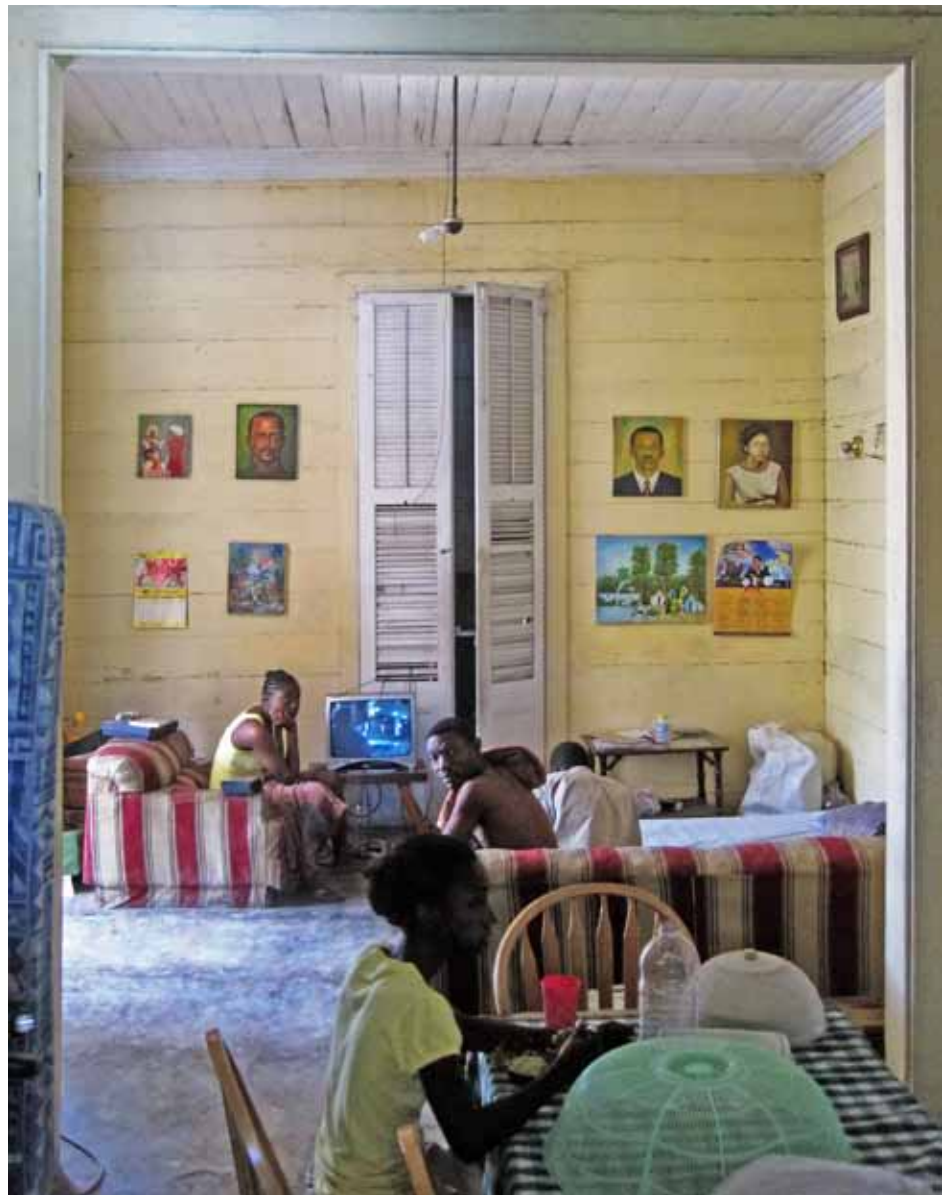
FIGURE 61 A typical interior of a Gingerbread house with wood floors, horizontal wood boarding on the walls, and wood board ceilings.
