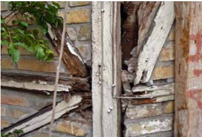
FIGURE 67 Rot of timber frame members at corner of colombage house at 32 Lamartiniere.
