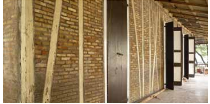
FIGURE 38 Colombage with brick and lime mortar infill at 30 Lamartiniere.
