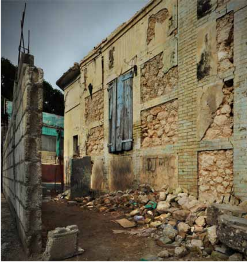
FIGURE 45 left: Wall of a commercial building on Avenue Lemartiniere showing the characteristic layout of the mixed brick with rubble stone masonry found in many Gingerbread houses in Port-au-Prince. The brick piers and horizontal brick courses are crucial in restraining the walls from complete collapse. right: Interior view of wall of the Villa Castel Fleuri (see Figure 1) showing a rubble stone panel which has completely collapsed out from between the brick masonry piers. Notice the brick keys that had extended into the rubble stone panel.
