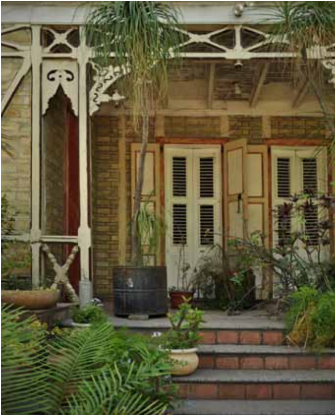
FIGURE 36 79 Avenue Christophe showing colombage with brick infilling.
