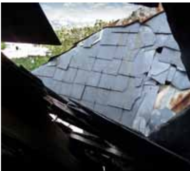
FIGURE 57 Original, thin slate roofing at 14 Avenue John Brown.
