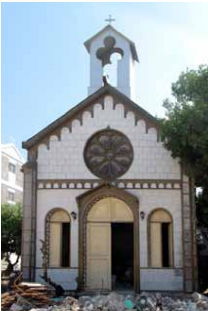
FIGURE 132 This small chapel next to the Cathedral has the same surface-applied steel reinforcement system as the Saint Louis de Gonzague Chapel and fared very well in the earthquake.”
