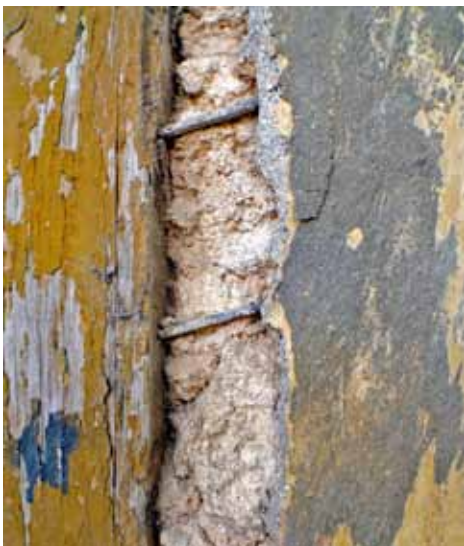
FIGURE 43 Nails help hold the earthen infill.
