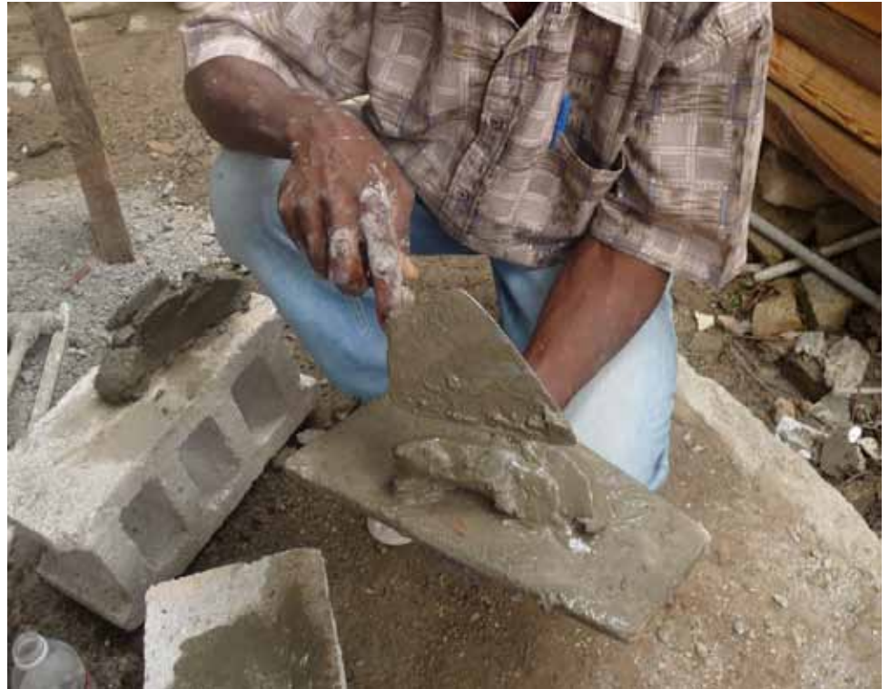
FIGURE 135 Well-intentioned but improper repairs with cement mortar in brick work ( left and center ), and cement plaster for colombage infill ( right ). Lime mortar and lime plaster should be used.
