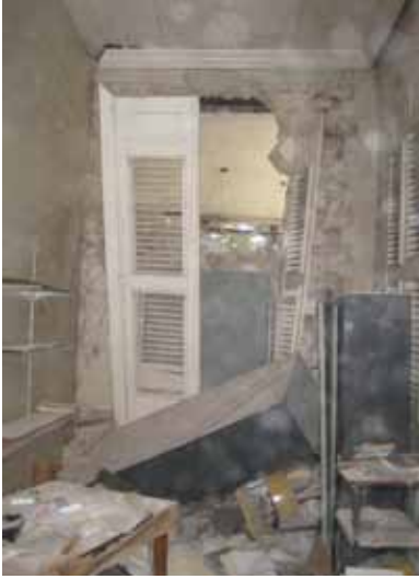
FIGURE 69 Hole in the masonry wall of Castel Fleuri caused by a concrete vault constructed in the exterior side and adjacent to this wall.
