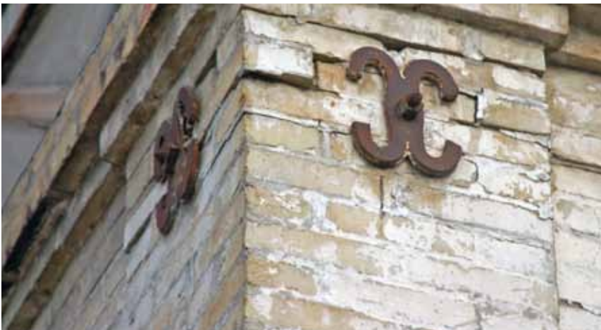
FIGURE 26 View of decorative end plates at the corner of this brick structure indicate horizontal ties along each wall of the intersect.
