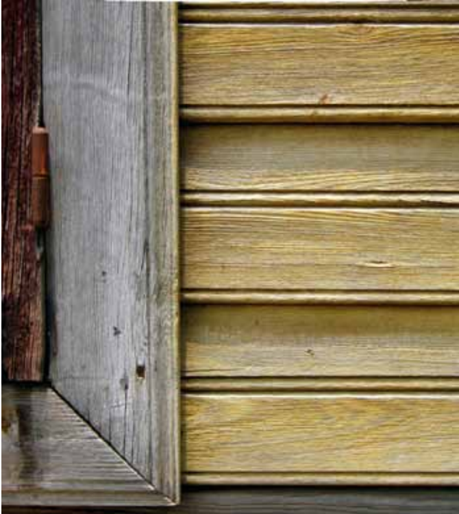
FIGURE 33 Some colombage houses have wood sheathing on the exterior as well as the interior
