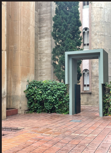
FIG. 5 Entrance to La Fábrica, 2022. (Photograph by author)
