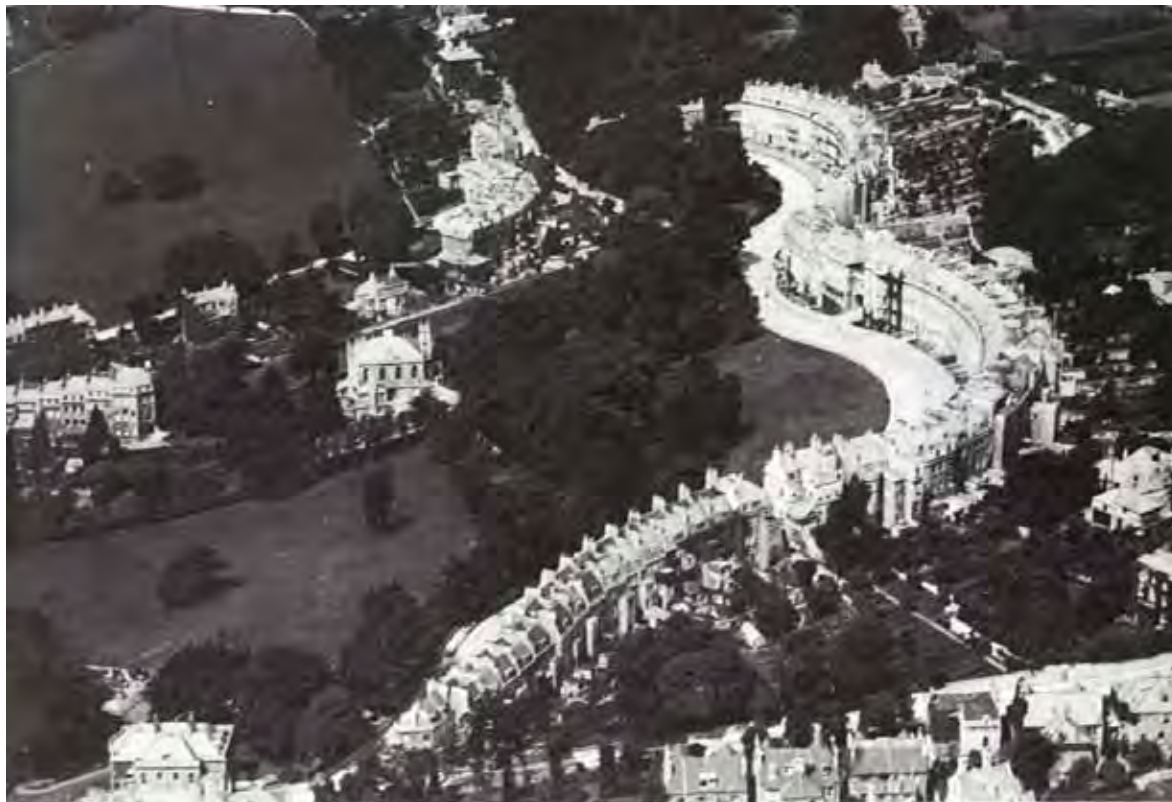
83. Lansdowne Crescent, Bath, 1794. Its serpentine windings follow the contours of the site.
