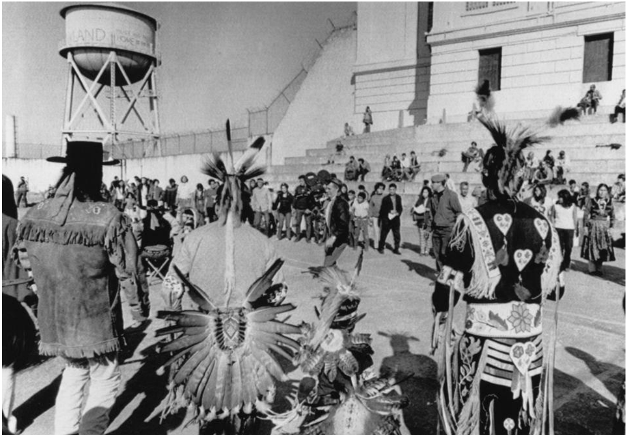
Occupants on Alcatraz Island, gather in front of the main cell block with the island's water tower ... [+]
