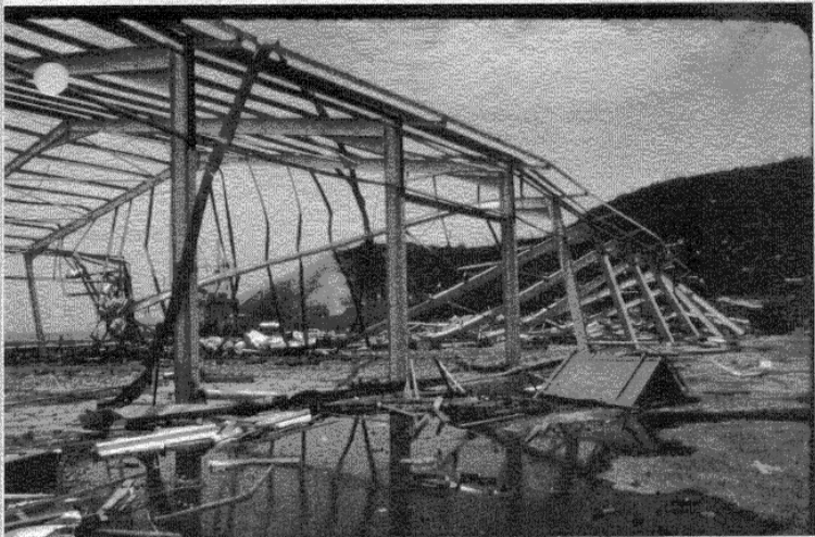
Photo 2 - Dramatic and total destruction of large, steel, portal-frame building (David)
