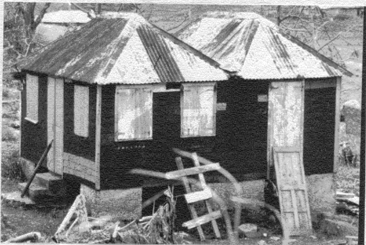
Photo 12 - The very favourable geometry saved this very modest house from any damage (Hugo)
