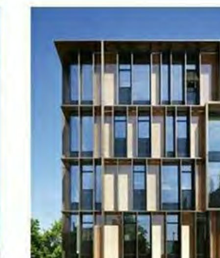
CW - 02 CURTAIN WALL WITH SHADING
