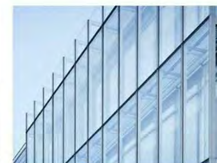
CW - 01 A UNITISED GLASS CURTAIN WALL
