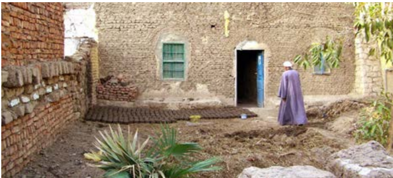
Mudbrick fabrication in the yard of a Fathy building now under renovation
