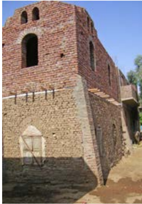
Reconstruction in Fathy style reusing ground floor earthen materials and fired brick above
