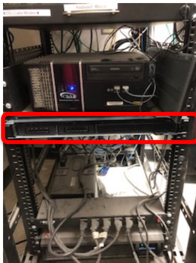
Shows server is installed in slot 12
