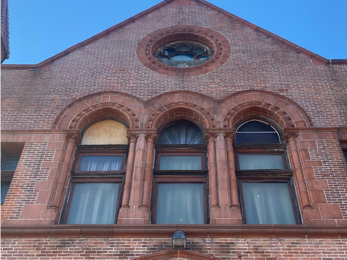
Figure 7. Damage to current windows on east facade (Photograph by author, 2021.)
