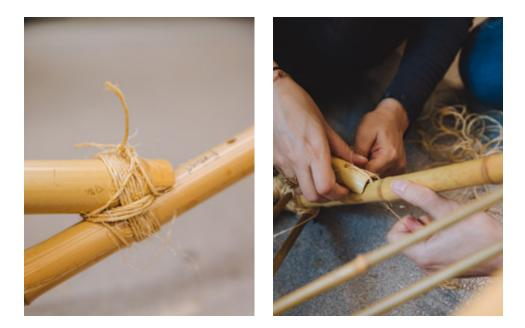
Figure (2) + (3): Lashing the fisheye joint
