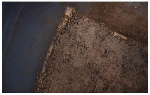
Figure (6): Mixture 04 is added (Medium sieved soil, sand and long straw)
